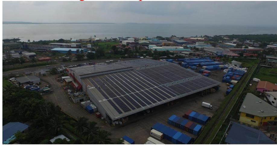
1.1MW solar system is equivalent in size to about 200 residential systems, consisting of over 3,860 solar panels. Producing 1,408,000 Kilowatt hours of energy per year, the system will save 974 tons of CO2 annually. Equivalent of saving 414,722 litres of diesel per year, or avoiding 3,730,751 car kilometres driven annually or planting 24,964 trees.
